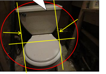
HOLES ON BATHROOM WALLS AND TOILET BOWL NOT LEVEL CLOTHING STORE
