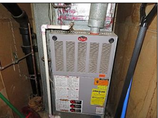
HEATING SYSTEM; WEATHER KING brand with A/C, natural gas type
