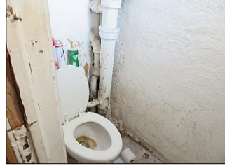
1/2 BATHROOM; Wooden doors- vinyl floor tiles- wooden sash windows- light fixtures.
