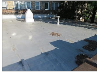
ROOFING SYSTEMS- MODIFIED BITUMEN - Steel gutters and down spout - roof tiles - concrete block and brick exterior chimney walls-
