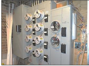
ELECTRICAL SYSTEMS OVERHEAD SERVICE DROP INLET WIRES - 800 Amperes - 12- 240 volts - 1 phase - step down to 100 amperes per unit - breaker type; located on each unit
