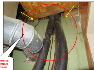
MISSING 1/2" TYPE DRAIN PIPES; UNIT 2 S
