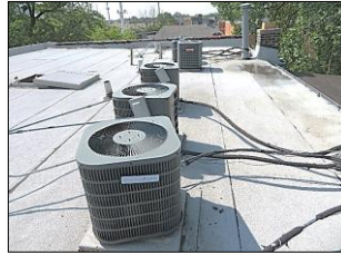
Sample pictures of HEATING & COOLING SYSTEMS: Individual force air furnace systems with A/C units - RHEEM brand, capacity on each unit - 75,000 B T U - year model 2003 - 2004; located on each unit
