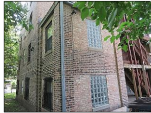
Sample pictures of EXTERIORS, FRONT EAST, SOUTH EAST/NORTH WEST & REAR WEST ELEVATION: Brick exterior- concrete walkway- steel gate and fences- thermal pane and glass block windows - rear wooden deck- light fixtures- cameras- flat roof with steel gutters and down spouts- rear steel gate open parking.
