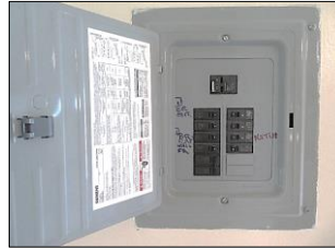
ELECTRICAL SYSTEMS OVERHEAD SERVICE DROP INLET WIRES - 800 Amperes - 12- 240 volts - 1 phase - step down to 100 amperes per unit - breaker type; located on each unit
