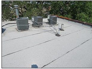
Sample pictures of ROOFING SYSTEMS: Flat roof - Modified Bitumen - tile copping- gutters and down spout; roof hatch opening located on common stairs top floor ceiling - GOOD / FAIR CONDITION
