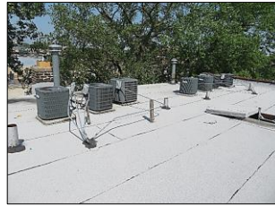
Sample pictures of ROOFING SYSTEMS: Flat roof - Modified Bitumen - tile copping- gutters and down spout; roof hatch opening located on common stairs top floor ceiling - GOOD / FAIR CONDITION
