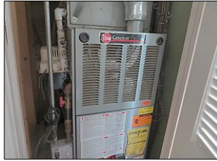
Sample pictures of HEATING & COOLING SYSTEMS: Individual force air furnace systems with A/C units - RHEEM brand, capacity on each unit - 75,000 B T U - year model 2003 - 2004; located on each unit
