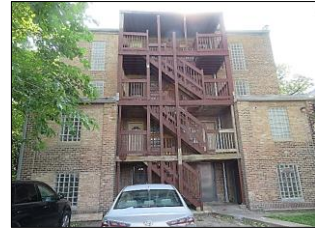
Sample pictures of EXTERIORS, FRONT EAST, SOUTH EAST/NORTH WEST & REAR WEST ELEVATION: Brick exterior- concrete walkway- steel gate and fences- thermal pane and glass block windows - rear wooden deck- light fixtures- cameras- flat roof with steel gutters and down spouts- rear steel gate open parking.
