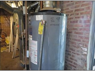
WATER TANK HEATER: RICHMOND brand - model # T82-156 - serial # CQ042BURIG0205G02059 - capacity 82 U.S. gallons - approximate year - 2-9-93; located; BASEMENT AREA
