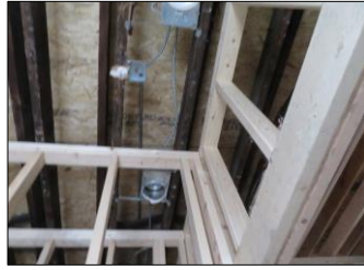
NEW DUCT WORKS, ROUGH PLUMBING AND ELECTRICAL SYSTEMS
