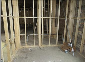
NEW ROUGH ELECTRICAL SYSTEMS ON 3RD FLOOR
