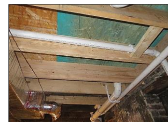
NEW PVC PIPES AND DUCT WORKS ON BASEMENT AREA
