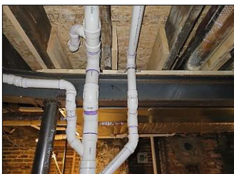
NEW ROUGH PVC PLUMBING SYSTEMS ON BASEMENT AREA
