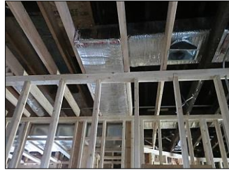
NEW DUCT WORKS AND REPLACEMENT OF WOODEN CEILING JOIST
