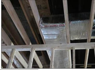
REPLACEMENT OF NEW WOODEN CEILING JOIST
