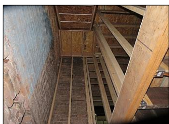
NEW STAIR HOLES/ SPACE TO BASEMENT LEVEL AND STAIRS TO 1ST FLOOR UNITS COMMON AREA
