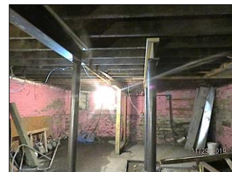
NEW STEEL BEAMS, COLUMNS AND CONCRETE FOOTINGS ON BASEMENT AREA
