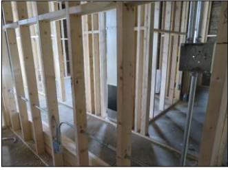
NEW DUCT WORKS, ROUGH PLUMBING AND ELECTRICAL SYSTEMS
