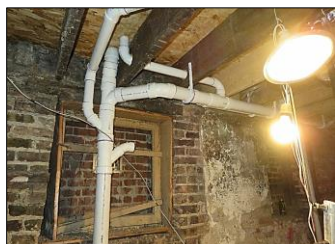
NEW ROUGH PVC PLUMBING SYSTEMS ON BASEMENT AREA
