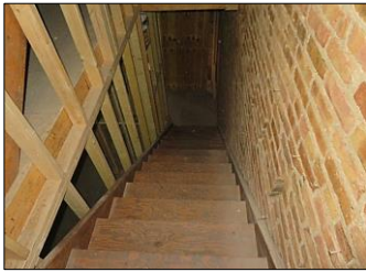
STAIRS TO 2ND FLOOR
