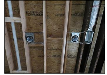
NEW DUCT WORKS AND REPLACEMENT OF WOODEN CEILING JOIST
