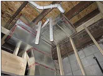
FINISHED DUCTWORKS AND WOOD BEAMS ON UTILITY ROOM AND MIDDLE REAR HALLWAYS
