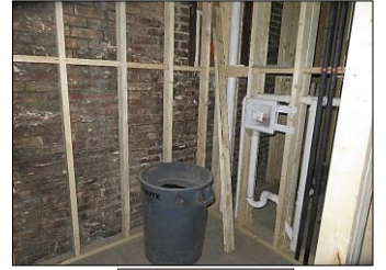
LAUNDRY ROOM/ UTILITY ROOM
