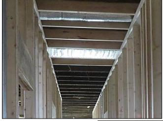
REPLACEMENT OF NEW WOODEN CEILING JOIST
