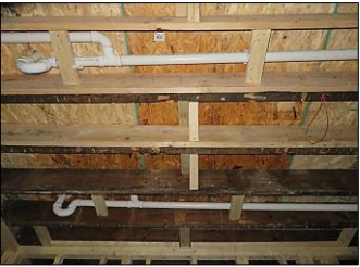
SAMPLE PICTURES OF ROUGH PVC PLUMBING SYSTEMS
