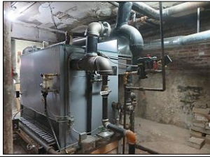
HEATING SYSTEMS: Boiler / Steam radiators - gas type - PEARLESS Brand - Model # 2114-12-S-1, SERIAL # 740983-2018-612 - CAPACITY - 2,310,000 BTU YEAR MANUFACTURED 2016 - Located on basement area.
