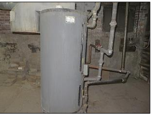
WATER TANK HEATERS: RUUD brand - Gas type - MODEL # G76-200-1 - SERIAL # A201814576 - CAPACITY - 74 US GALLONS - YEAR MANUFACTURED 2018 # 2 TANK - RUUD brand - Gas type - MODEL # RF76-200 - SERIAL # 08920070081 - CAPACITY 76 U S GALLONS - YEAR MANUFACTURED 2007
