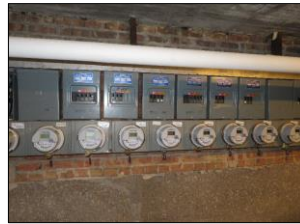
ELECTRICAL SYSTEMS: OVERHEAD service drop inlet wires - 600 Amperes main service - step down to 100 & 65 Amperes per unit - breaker type - located on basement area.
