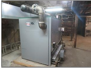
HEATING SYSTEMS: Boiler / Steam radiators - gas type - PEARLESS Brand - Model # 2114-12-S-1, SERIAL # 740983-2018-612 - CAPACITY - 2,310,000 BTU YEAR MANUFACTURED 2016 - Located on basement area.
