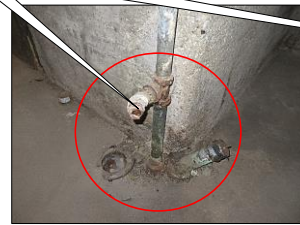
MISSING DI - ELECTRIC UNION/ RUSTED AND CORRODED WATER PIPES ON BASEMENT AREA; TAKEN PICTURES ARE SAMPLE PICTURES ONLY, PLEASE CHECK ENTIRE BASEMENT PLUMBING SYSTEMS
