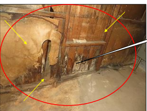
WATER LEAKING ON LAUNDRY SINK DRAIN PIPES, LAUNDRY ROOM
