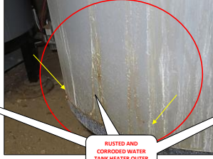
RUSTED AND CORRODED WATER TANK HEATER OUTER RIM
