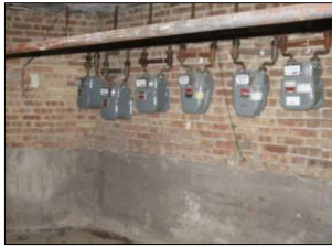
Sample pictures of UNIT GAS METERS : Located on basement area
