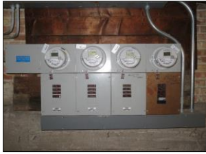
Sample pictures of UNITS ELECTRICAL SYSTEMS: BREAKER TYPE - 100 & 65 AMPERES PER UNIT; LOCATED ON BASEMENT AREA
