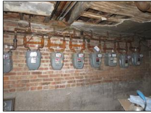
Sample pictures of UNIT GAS METERS : Located on basement area
