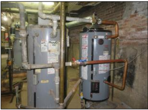
WATER TANK HEATERS: RUUD brand - Gas type - MODEL # G76-200-1 - SERIAL # A201814576 - CAPACITY - 74 US GALLONS - YEAR MANUFACTURED 2018 # 2 TANK - RUUD brand - Gas type - MODEL # RF76-200 - SERIAL # 08920070081 - CAPACITY 76 U S GALLONS - YEAR MANUFACTURED 2007
