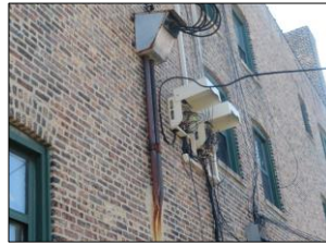
ELECTRICAL SYSTEMS: OVERHEAD service drop inlet wires - 600 Amperes main service - step down to 100 & 65 Amperes per unit - breaker type - located on basement area.
