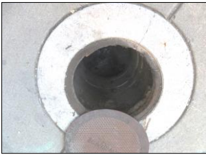
Sample pictures of CATCH BASIN: Good and clean condition
