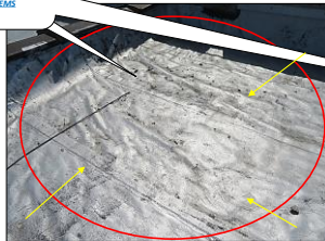
DAMAGED ROOF TILES AND BULGING ROOFING SYSTEMS ON DIFFERENT AREAS: TAKEN PICTURES ARE SAMPLE PICTURES ONLY, PLEASE CHECK THE ENTIRE ROOFING SYSTEMS
