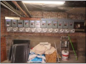
Sample pictures of UNITS ELECTRICAL SYSTEMS: BREAKER TYPE - 100 & 65 AMPERES PER UNIT; LOCATED ON BASEMENT AREA
