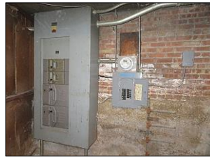
ELECTRICAL SYSTEMS: OVERHEAD service drop inlet wires - 600 Amperes main service - step down to 100 & 65 Amperes per unit - breaker type - located on basement area.
