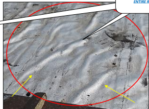
DAMAGED ROOF TILES AND BULGING ROOFING SYSTEMS ON DIFFERENT AREAS: TAKEN PICTURES ARE SAMPLE PICTURES ONLY, PLEASE CHECK THE ENTIRE ROOFING SYSTEMS
