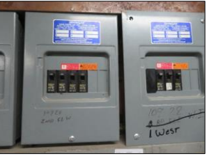
Sample pictures of UNITS ELECTRICAL SYSTEMS: BREAKER TYPE - 100 & 65 AMPERES PER UNIT; LOCATED ON BASEMENT AREA
