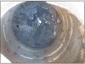
Sample pictures of CATCH BASIN: Good and clean condition
