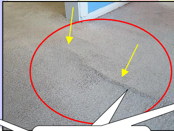
SAMPLE PICTURES OF LOOSE DAMAGED AND BULGING CARPET COVERING
