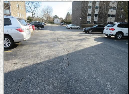
OPEN PARKING LOT
