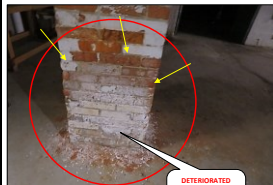
DETERIORATED BRICK COLUMN ON BASEMENT AREAS
