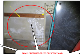
SAMPLE PICTURES OF EFFLORESCEANCE AND BUCKLING CONCRETE WALLS ON BASEMENT AREAS; TAKEN PICTURES ARE SAMPLE PICTURES ONLY, PLEASE CHECK THE ENTIRE BASEMENT WALLS.
