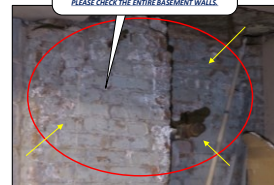
SAMPLE PICTURES OF EFFLORESCEANCE AND BUCKLING CONCRETE WALLS ON BASEMENT AREAS; TAKEN PICTURES ARE SAMPLE PICTURES ONLY, PLEASE CHECK THE ENTIRE BASEMENT WALLS.
