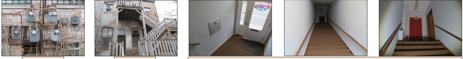
GAS METERS REAR WOODEN PORCH FRONT COMMON STAIRS & LOBBY (13125 ENTRY): Steel doors with glass panes - carpet wooden stairs with carpet coverings - light fixtures - mailboxes - drywalls - radiator heater
