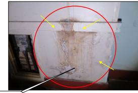
WATER DAMAGED ON BASEMENT WALLS AND CEILING
