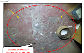
DAMAGED AND WEAK FLOORS 13125 - 2 R
