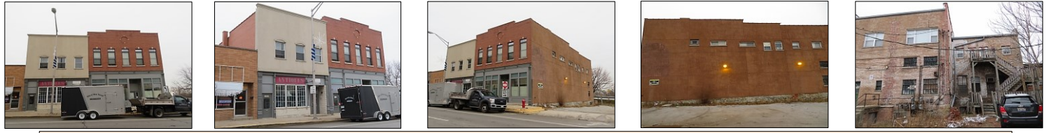
Sample pictures of EXTERIORS; Front West, North West, South West, South and rear East Elevation: Brick, wooden and stucco exteriors - light fixtures - thermal and casement windows - wooden porch - flat rubber roofs with steel gutters and down spout - City poured concrete walkway - vacant lot on South sections of the property.
